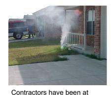
work looking for cracks in our sewerage system. Appearance of smoke above ground indicates a likely location for storm water entering and overloading the system. Ross is monitoring
